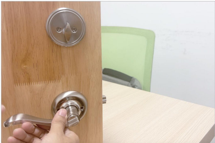
9. Install the interior parts: Ensure the interior knob H is centered over the positioning nut before tightening.
