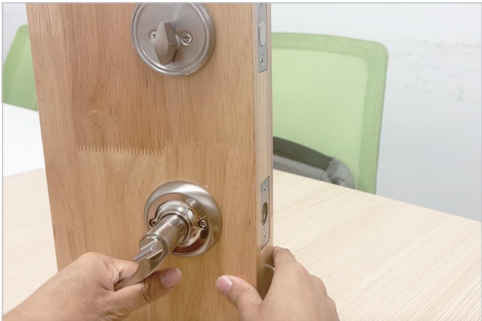
11. Make sure you can turn the knob and key easily without any sticking.
