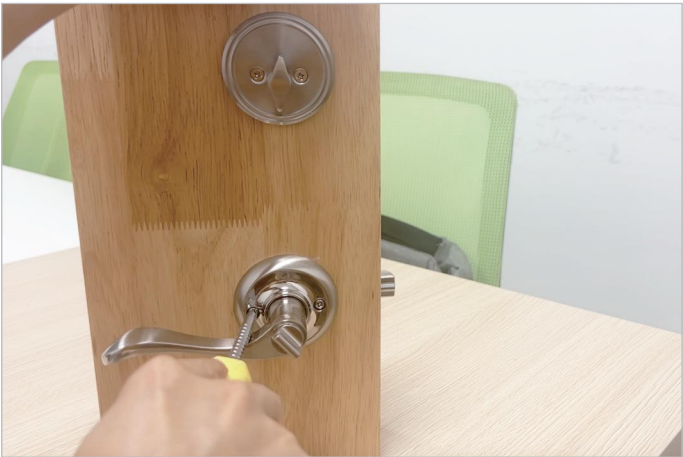
10. Install the interior parts: Secure the knob H with screw N.
