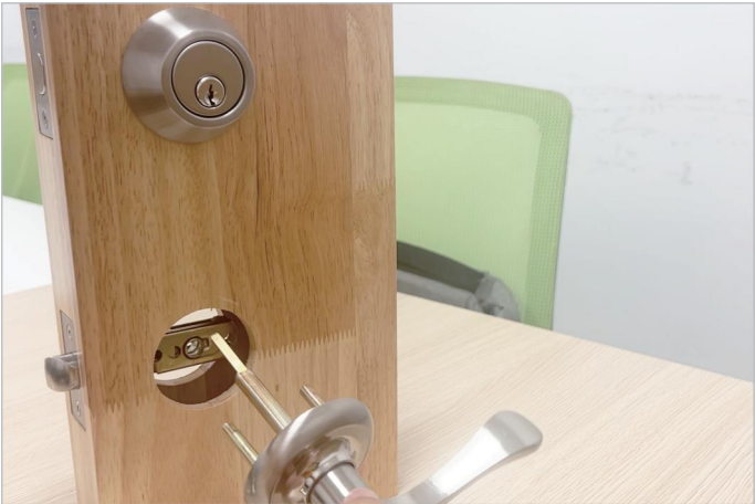
8. Install the exterior parts: Put on the knob G and line it up with the hole in the latch bolt.
