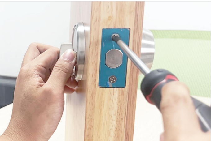
6. Turn the screw on the face plate to make the lock feel smoother when you turn it.
