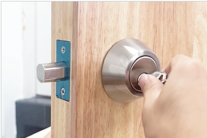
5. Make sure you can turn the thumbturn and key easily without any sticking.
