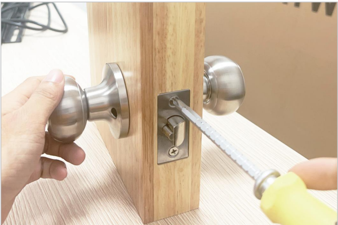
12. Turn the screw on the face plate to make the lock feel smoother when you turn it.
