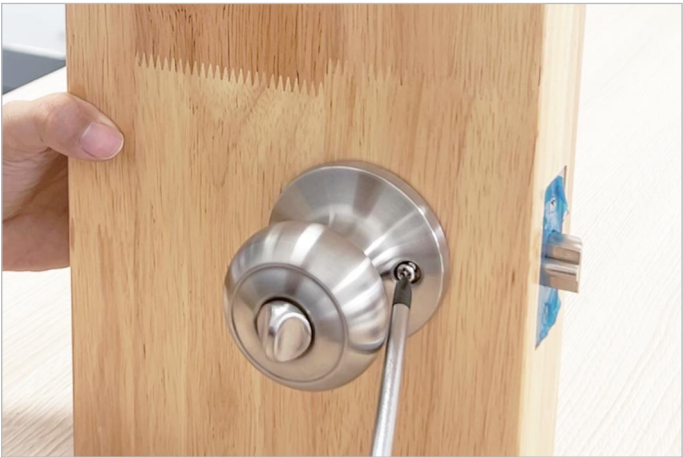
10. Install the interior parts: Secure the ball knob H with screw O.
