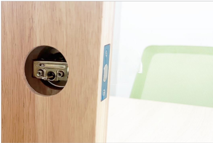
3. Install the interior parts: Ensure the lock tongue is retracted and the flat rod is in a horizontal position.
