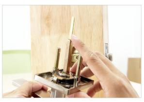
2. Install the exterior parts: Put on the knob A and line it up with the hole in the latch bolt.
